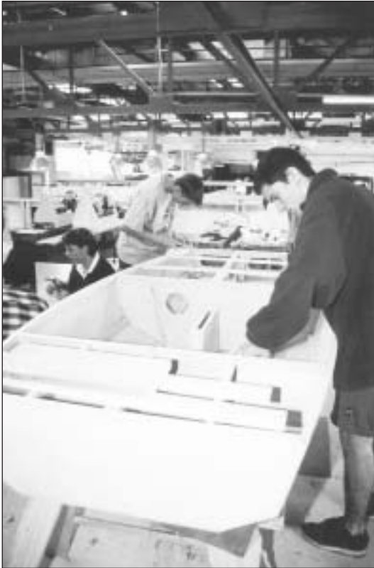
3 UNITEC School of Boatbuilding workshop
