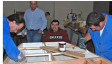
Sealing the inside before gluing on the deck.
