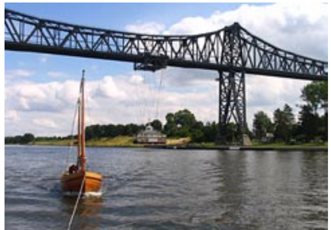
Numerous bridges and ferries - this 'ferry' suspended on cables beneath the bridge.
